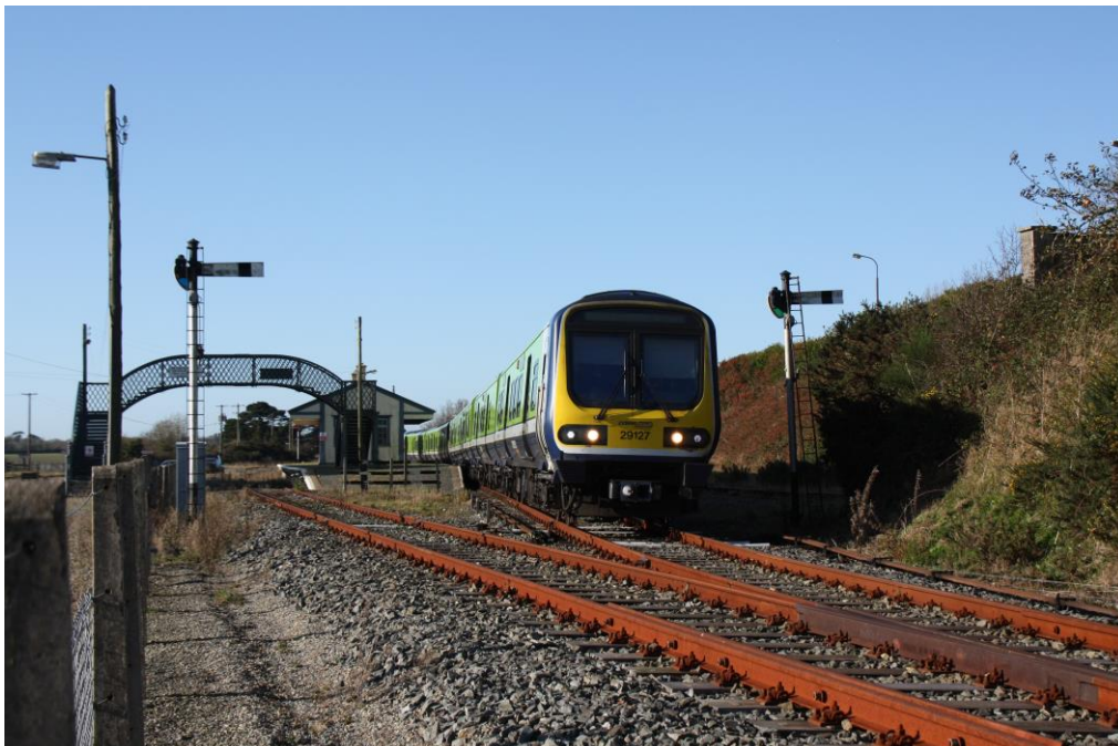
Figure 49 - IE Unit during Stock Transfer at Wellingtonbridge Station
